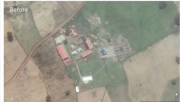
Example 1: Demolition of Mosque
